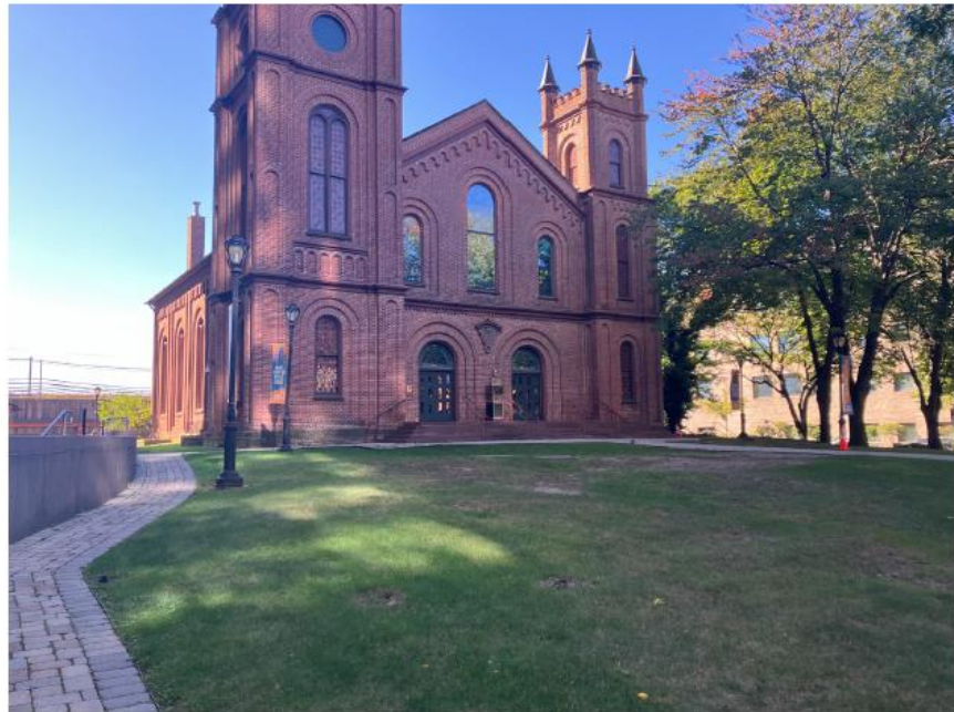
View from NE area of site - Existing
